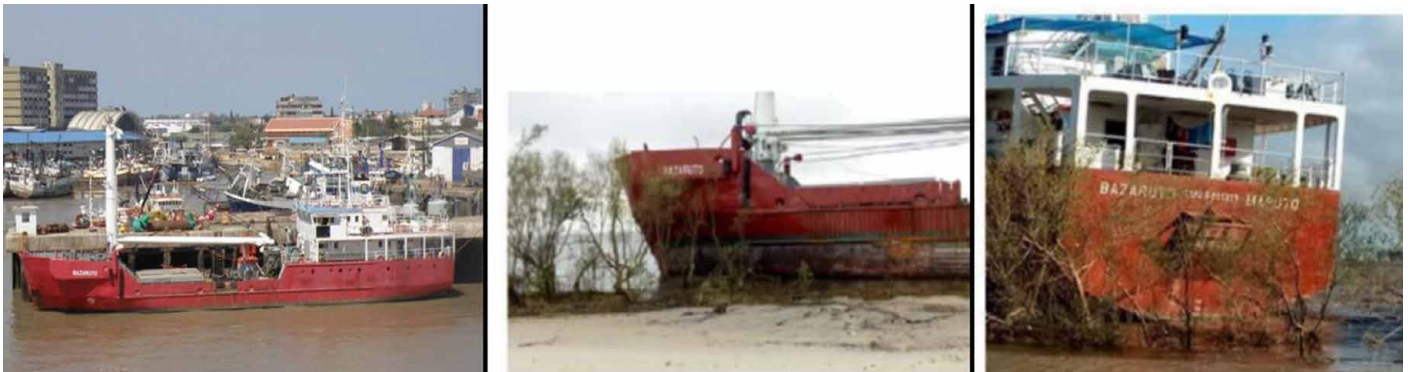
Fig. 3 Mozambique Buoy Tender 'Bazaruto', before (left) and after (centre, right) 2019 Cyclone Idai. Images credit E. Tarasov, MarineTraffic.com (left) and The International Hydrographic Review (centre, right). (Harris, 2002), a predecessor to the Songimvelo co-management project, Eastern Cape Province, South Africa. Images courtesy World Resources Institute.
