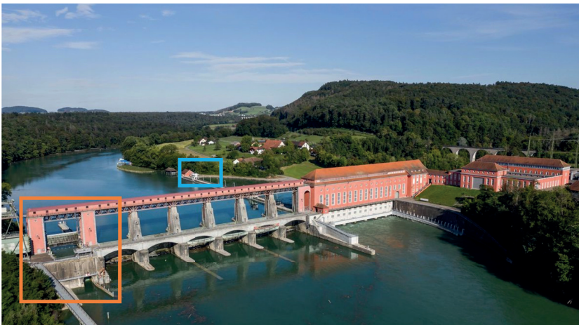
Fig. 3 The Hydropower plant in Eglisau: The water lock (orange) and the water filter (blue) in the inlet basin.
